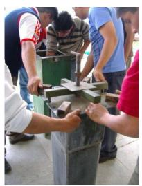
Figure 4: Removal of the concrete filter from the metal mould. Photo: Soluciones Prácticas.
